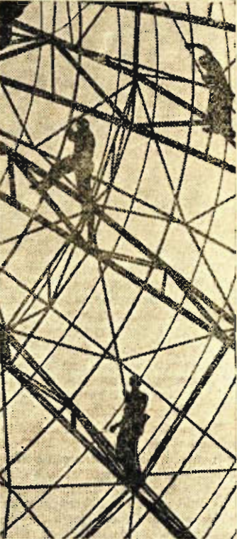
RESEMBLING CREATURES caught in a huge spider web, workers at Akron, O. construct radar tracking antenna for air force missile warning system.
