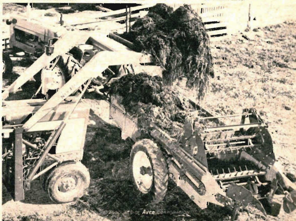
POPULAR SIZE CYLINDER/PADDLE. For fine shredding and controlled, uniform spreading. This ruggedly built 145-bushel New Idea cylinder/paddle spreader is ideal for larger dairy and livestock farmers.
