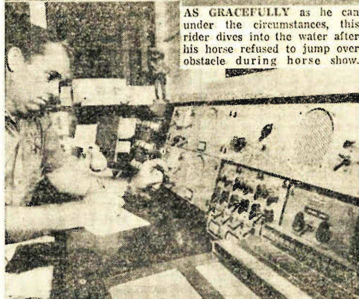
PUSHBUTTON JAIL in Logan, Utah uses a Honeywell security console to electronically keep the prisoners locked up safely in their cells. One man can control whole jail from this unit.
