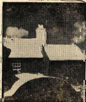
RAIN ROOF . . . This Bermuda house, built in 1705, shows some of the distinctive architecture of the island. The gleaming white roof, used to catch rainwater for the household, tops rough-hewn limestone block walls. The round-topped tank in foreground is used to store rainwater.
