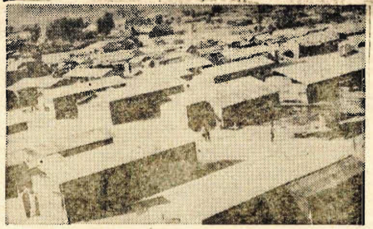
NEW VILLAGE . . . This is the rebuilt Catholic refugee village of Phuoc Quang, South Vietnam. When fire destroyed 160 houses, Navy Seabees came from nearby DaNang to assist villagers in restoration.
