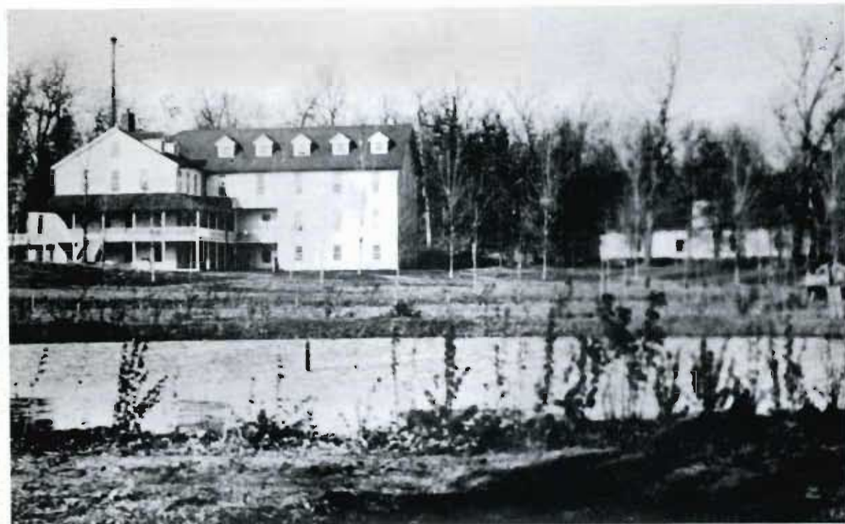
Photo shows Culver Park Assembly Grounds, 1889. At left, frame structure provides for dining room, administrative center, and 16 guest rooms, top floor. At right can be seen the Tabernacle, where 1889 Assembly Series was held.
