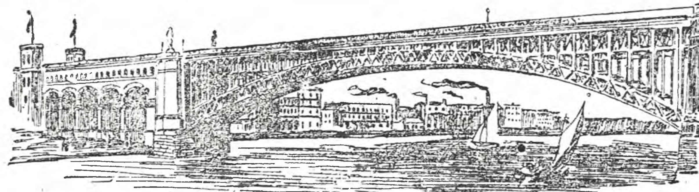
THE GREAT EADS BRIDGE OVER THE MISSISSIPPI RIVER.
