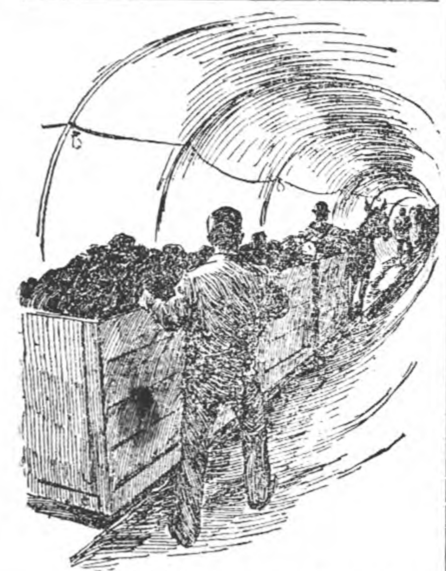
HAULING DIRT IN THE TUNNEL.
