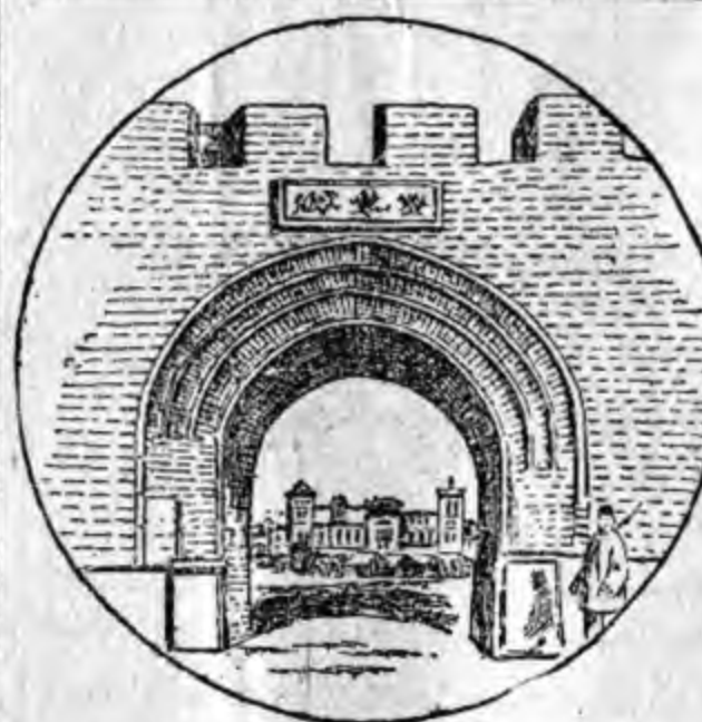
GATE OF THE TIEN-TSIN WALL.
