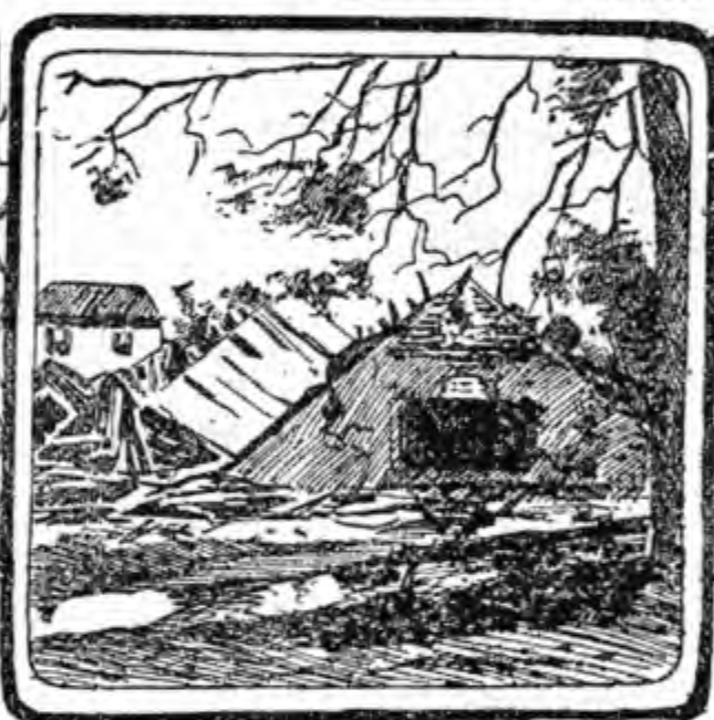
BUILDING BLOWN HALF A MILE.
