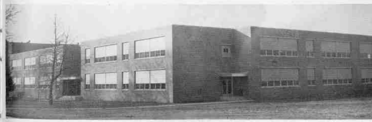
THE NEW ELEMENTARY BUILDING AS VIEWED FROM THE NORTHEAST CORNER
