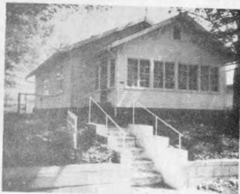
Culver - 910 Baker St. - Finished basement.
