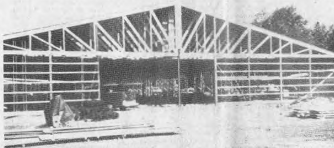
This is the site of the Shirt Shed, Inc., construction. The plant is planning a November opening and will employ approximately 150.
