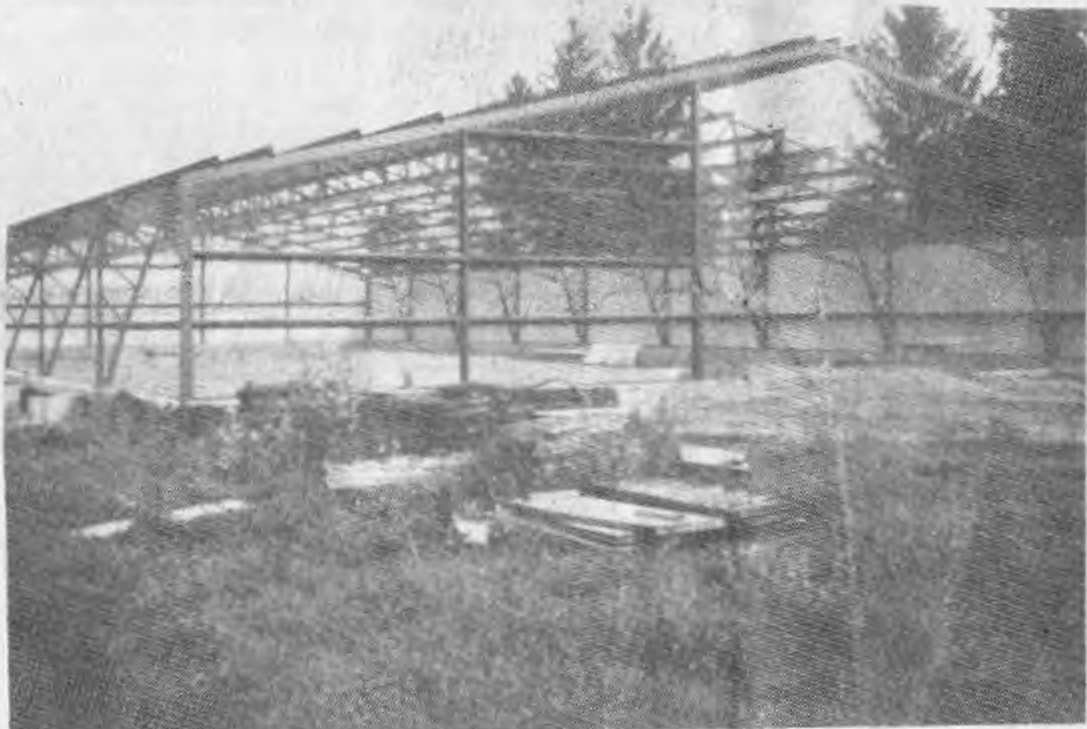
The new bowling alley being built by Camelot Universal Corp., is located on Highway 10 and 17 just west of the junction. Builders are trying for a late November opening.
