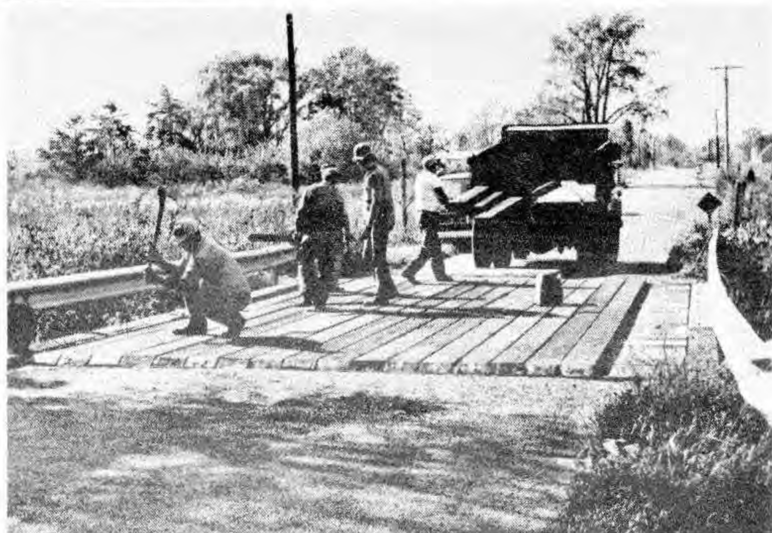
WORKING TOGETHER to repair a bad bridge are crews from both Starke and Pulaski Counties. This is the bridge on the extension of State Road 110 west of State Road 17 on the way to Ora. Often called the Fox Bridge (Because it was near where Fred Fox lived), the bridge had been in poor repair for months. Here, a crew from Pulaski County replaces the planking on Monday. Starke County crews were to repave the approaches on Tuesday, with the road scheduled to be open for traffic yesterday or today. CITIZEN photo
