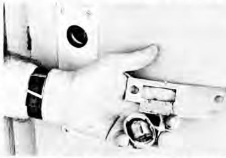
HOLDING THE BROKEN LOCK from his store door is Robert McKinnis, showing the way the
