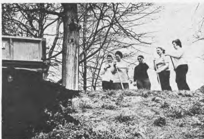
THE FIRST STEP in stopping the erosion is black dirt—lots of it! The dirt is used to fill in the gullies; it is then smoothed, the vetch is planted, and the planting is covered with straw and anchored to prevent wind erosion while the plants take root. Above, Jackie (Mrs. Larry) Berger, Rosaline (Mrs. James) Bonine, Lorraine (Mrs. Norman) DuMaine, Connie Overmyer and Linda (Mrs. John) Deery watch while a dump truck deposits a generous load of dirt in one of the gullies. CITIZEN Photo
