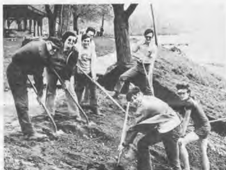
AND NOW, THE FUN BEGINS...Here's the part that separates the...well, whatever. This group is smoothing the dirt into the eroded areas to facilitate planting of the crown vetch. From left, the work crew consists of George Hopple, Kay (Mrs. Ronald) Tusing, Kevin Bonine, Nancy Thomas, Gary Connant, Georgie Hopple, and Jeff Thomas. CITIZEN Photo
