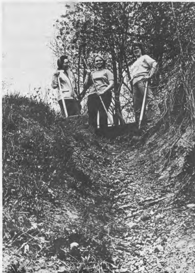
IT'S A LONG WAY DOWN—Members of the Maxinkuckee Junior Women's Club survey the task ahead of them...a gully caused by erosion of the embankment along the shore of Lake Maxinkuckee at the Town Park. The Junior Women spent last weekend filling several gullies such as this along the slope with black dirt and planting crown vetch in the areas to stop further erosion. As you can see from the pictures here, the job meant a long weekend's work and sore back muscles Monday, but Nancy (Mrs. Kenneth) Thomas, Connie (Mrs. Michael) Overmyer, and Mary (Mrs. Robert) Radawski don't seem to mind. CITIZEN Photo
