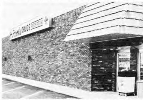
THIS NEW 7,000 square foot building has been erected at 103 South Ohio Street to house the new Hook's Drug Store in Culver. Opening ceremonies are scheduled for next Thursday, May 30th. See story to left. CITIZEN Photo
